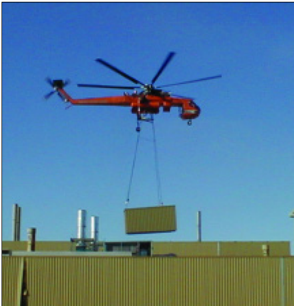
Fabrication & Installation, Intake Hood of an Air Supply House Project (above/below)
